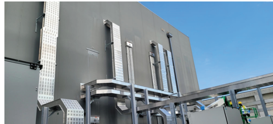
Image: Cable Bus Installation
