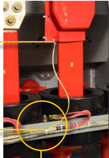
Figure 16 Safe Dielectric Routing Practices
