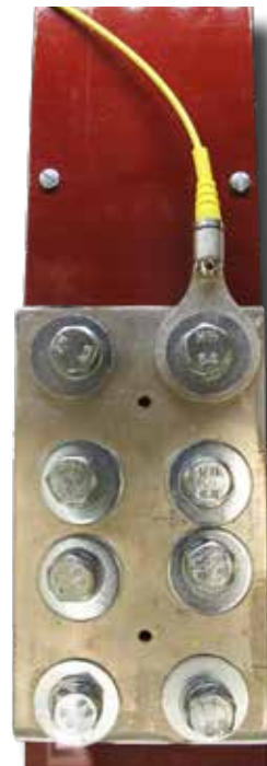
Figure 11 Correctly Installed Probe and Lug
