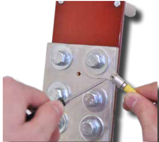
Figure 10 Secure Probe Tightening Allen Key
