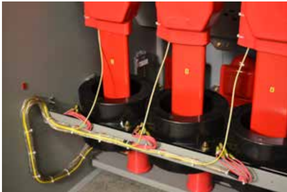
Figure 15 Completed Fiber Installation
