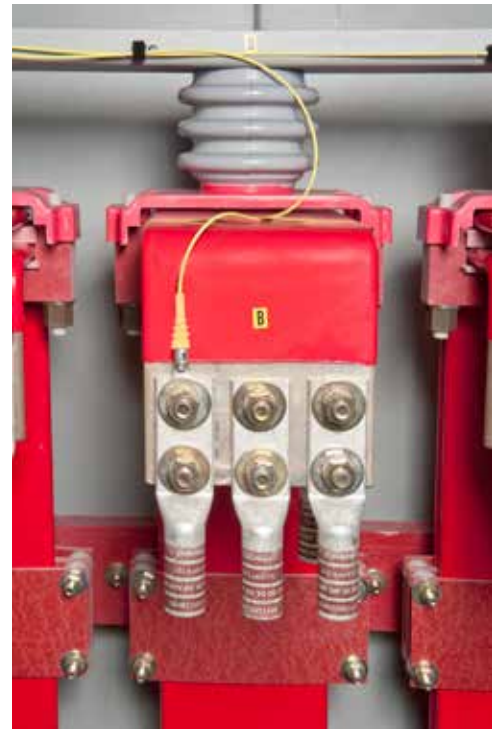
Figure 14 Tie-Wrap Being Secured Over Fiber
