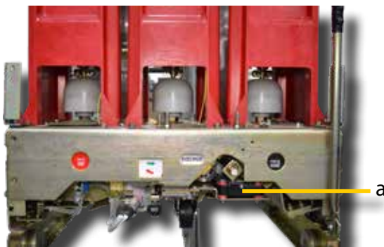
a. CBM Placement at front of Circuit Breaker with cover removed
