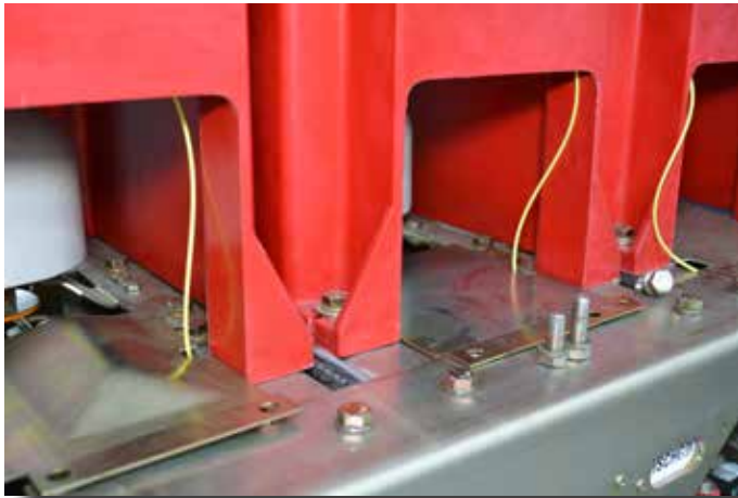
Figure 36 Fibers Terminate in CBM Unit
