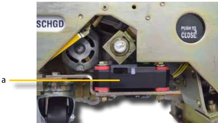
Figure 36 Fibers Terminate in CBM Unit
